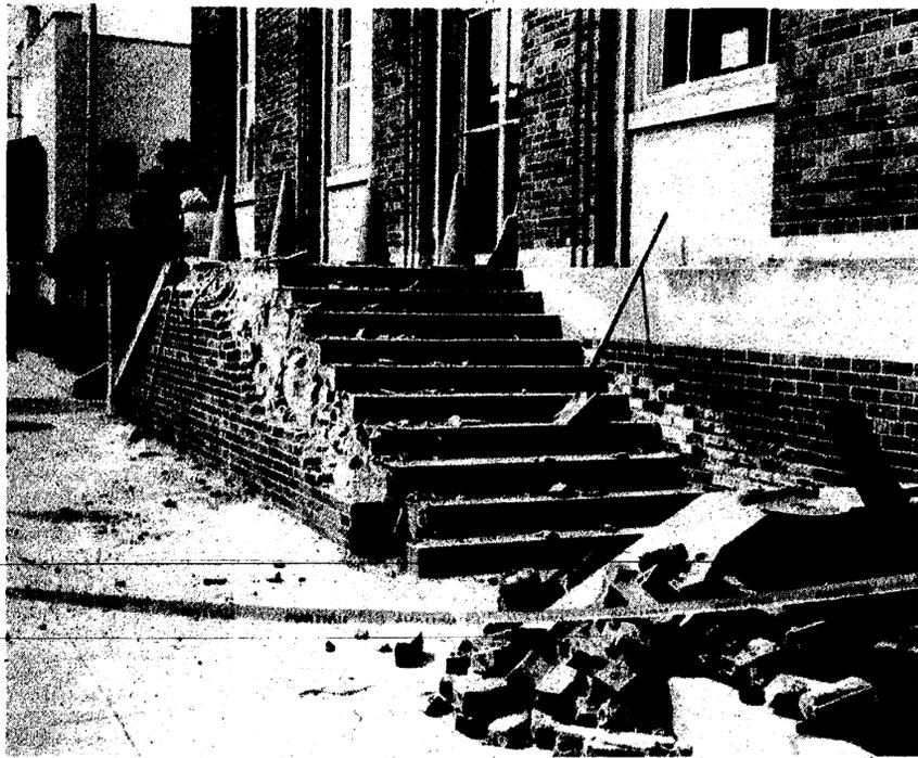
THE BRICK WALL AT THE FRONT of the steps at the Chelsea Post Office is being replaced. Water seeped behind the wall, causing it to crack. The wall was replaced about five years ago for a similar problem. Postmaster Larry Williams hopes the problem will be solved permanently this time.
